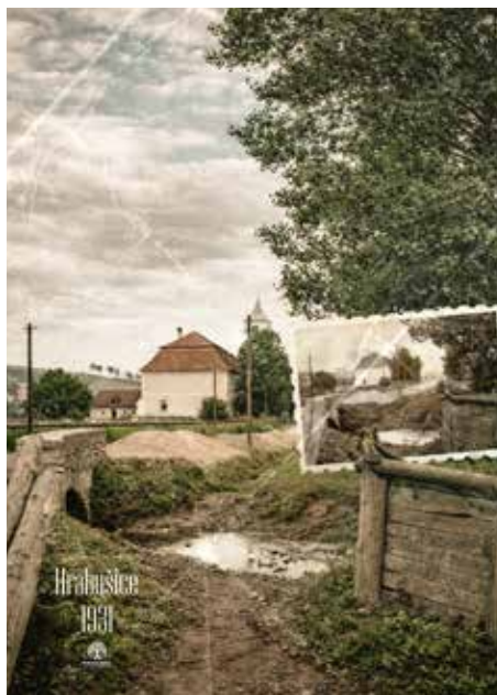
Hrabušice in 1931 and the old stone bridge, which no longer exists today.
